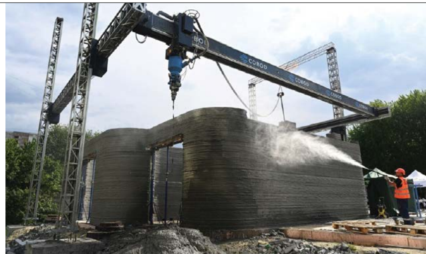
Printing nozzle at work in Lviv, Ukraine. (Image: www.rferl.org © Yurly Dyachyshyn, AFP)
