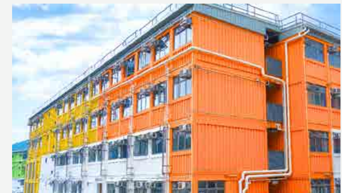
Transitional Housing Project at Fan Kam Road
