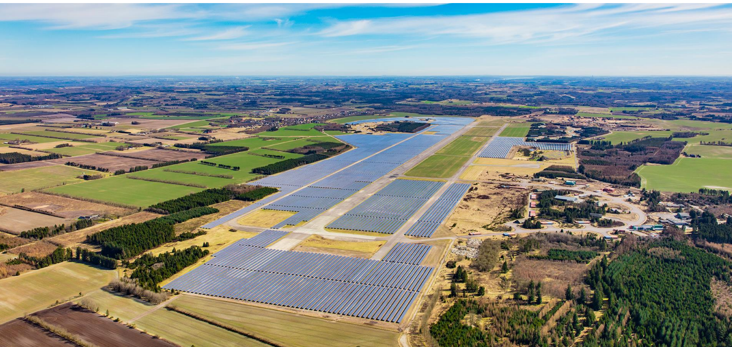
BeGreen's solar park, Vandel
