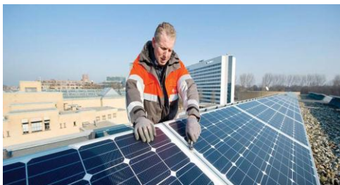
Installation/maintenance (e.g. solar PV, heat pumps)
