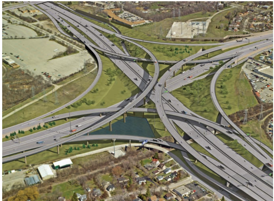
Models created for the construction of major projects now provide data for asset management throughout the life of the asset.
